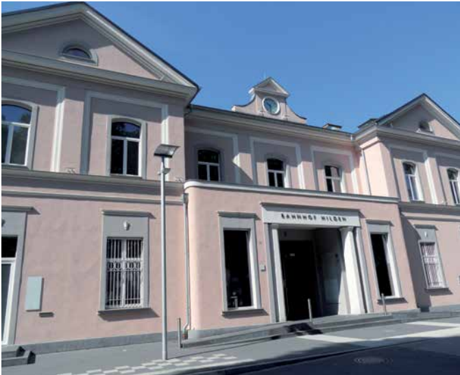
02 The advantages are evident especially for protected buildings: The easy installation preserves the historic structures.
